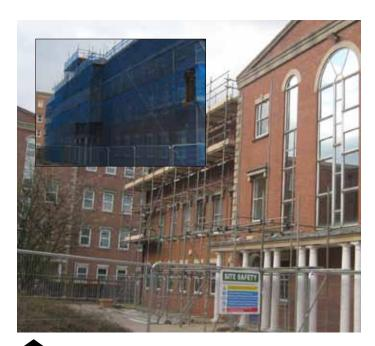
Structural failures to the facade of an office building in town centre required extensive scaffolding. Out of hours working and close co-ordination with the client allowed the works to proceed with the minimum of disruption for the busy office.
