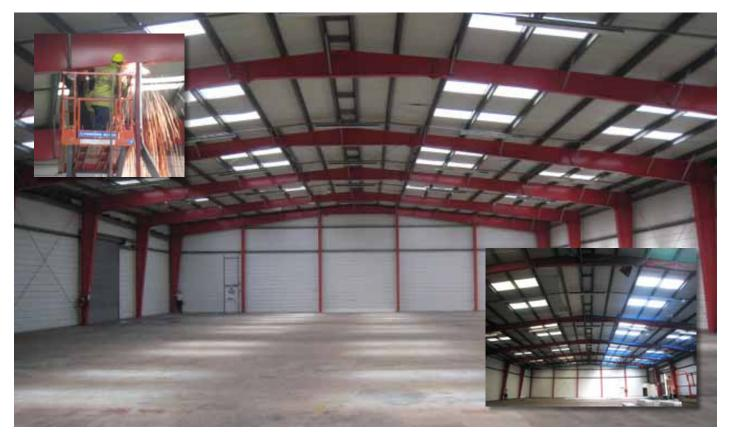
During the refurbishment of a recently vacated builders merchants in Daventry, roof repairs & light replacements required thrapeze safety netting to the entire structure.
